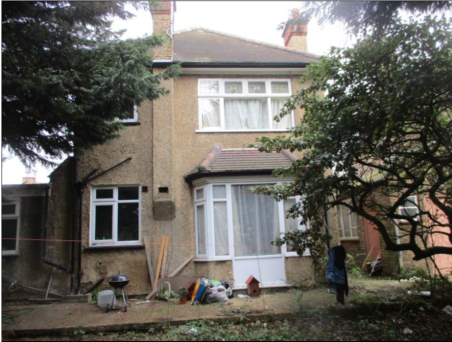
Rear Elevation of no. 9
