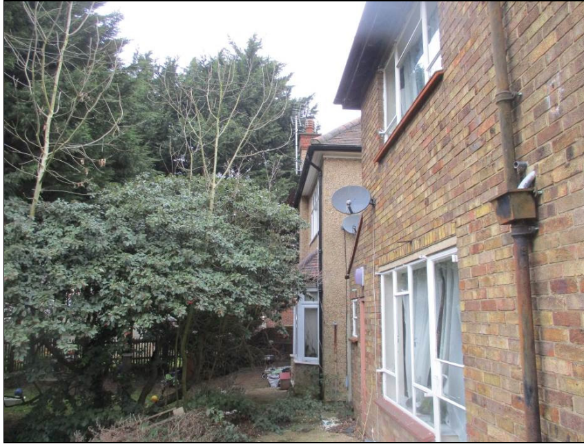
Rear elevations of no. 9 and 11
