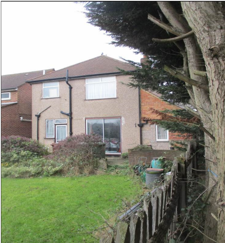
Rear of no. 7
