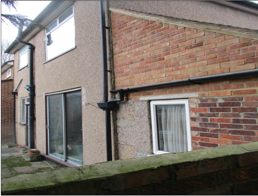
Rear of garage adjacent to boundary with no.9
