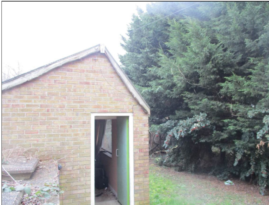
Rear outbuilding at no. 11
