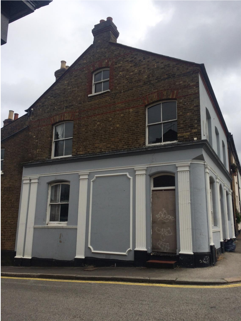
Figure 2 Side elevation of property
